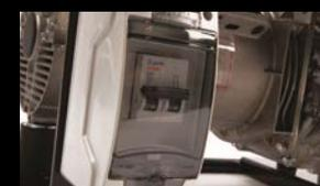
Our generators can optionally be equipped with this protection. In case of overcharge, the thermal circuit breaker will switch off directly, this ensures that both the alternator and the connected appliance will remain protected. This option detects a short circuit as well.
